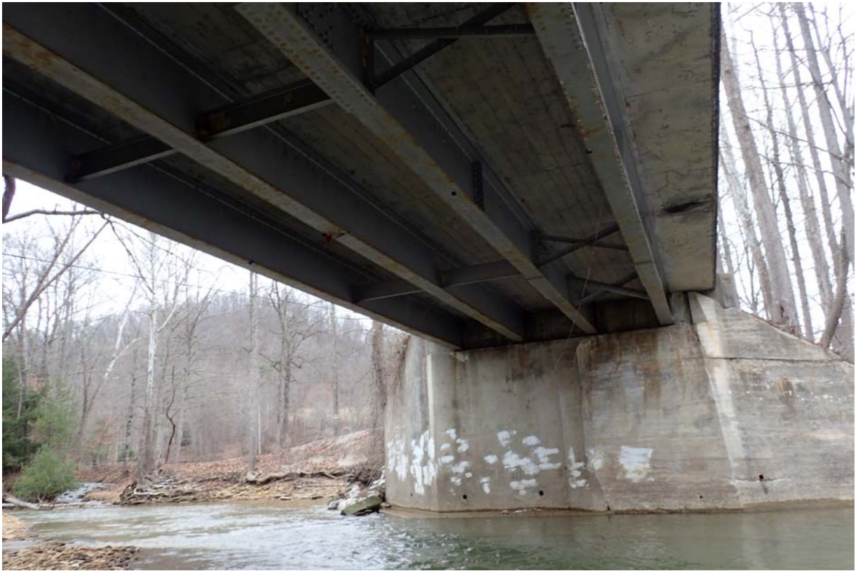
Typical view of the beams, deck underside, and abutment 2.
