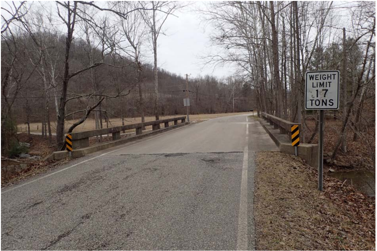
17 tons posting near abutment 1.
