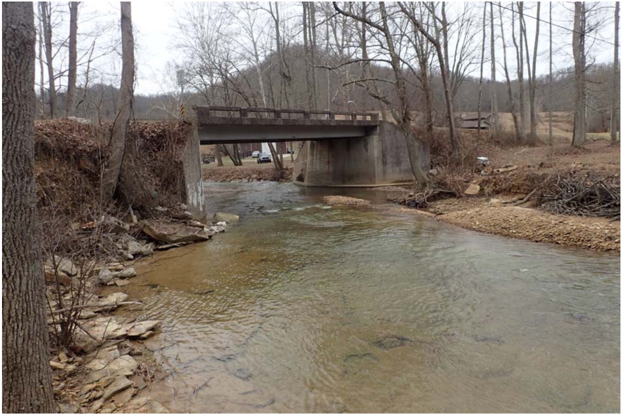
View from upstream.
