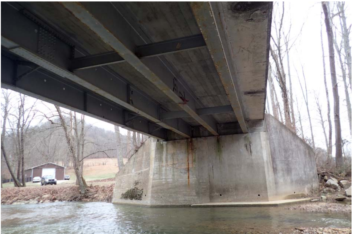
Typical view of the beams, deck underside, and abutment 1.
