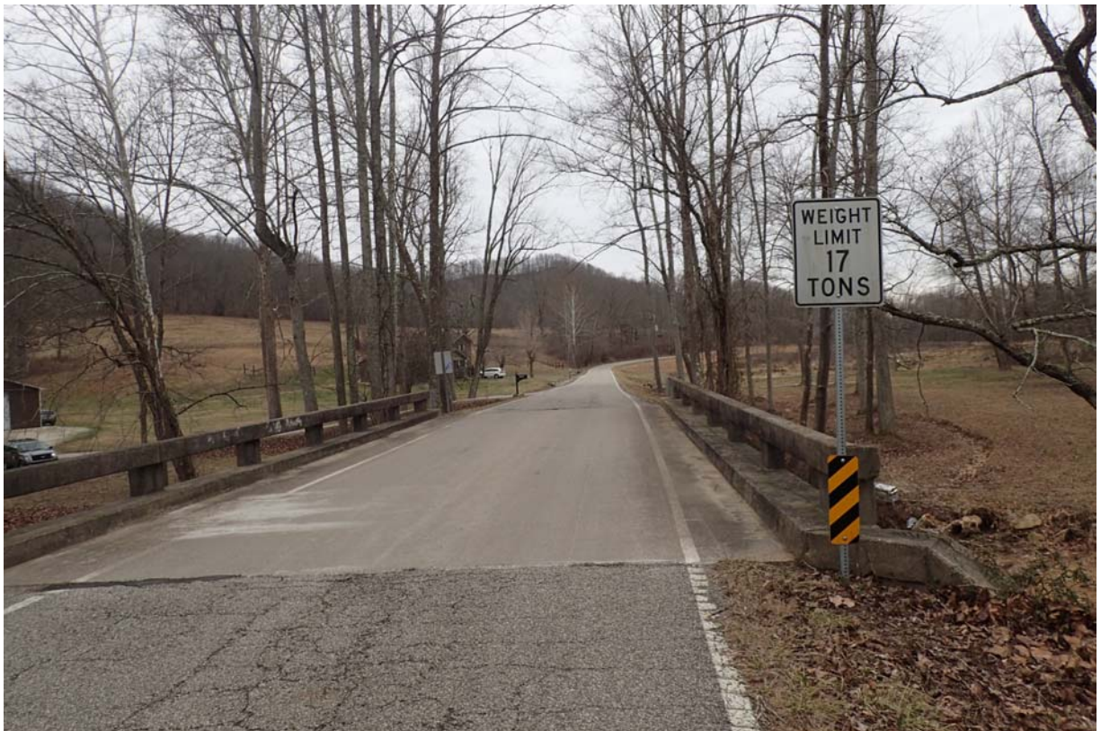
17 tons posting near abutment 2.
