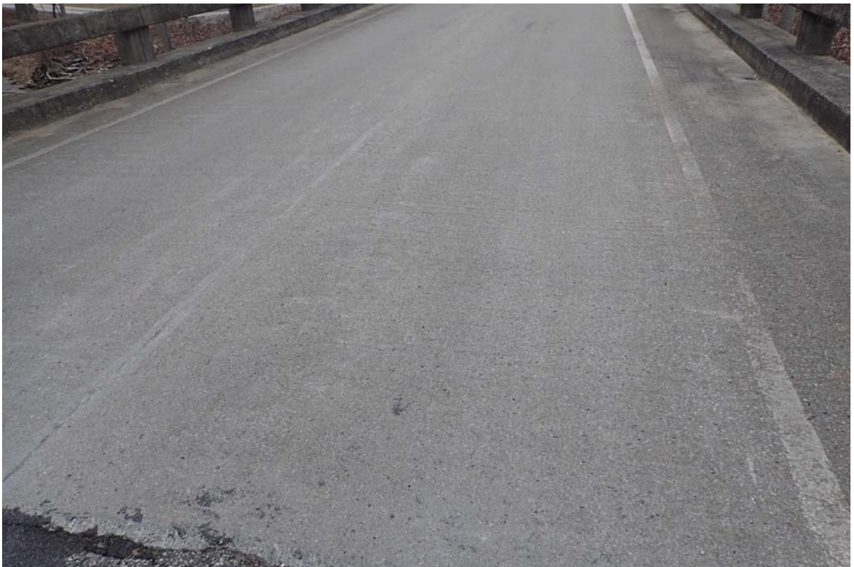
Typical view of the wearing surface.
