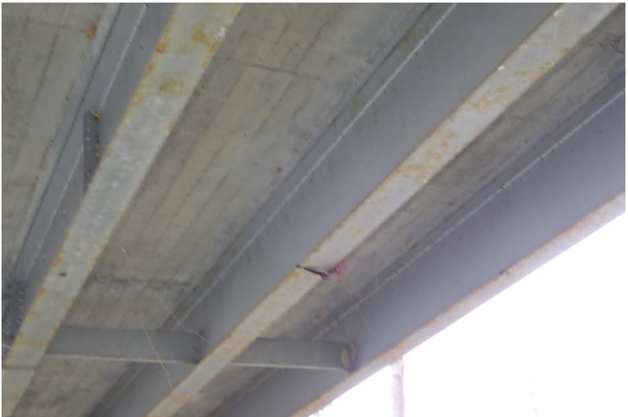
Typical view of the beams near midspan.
